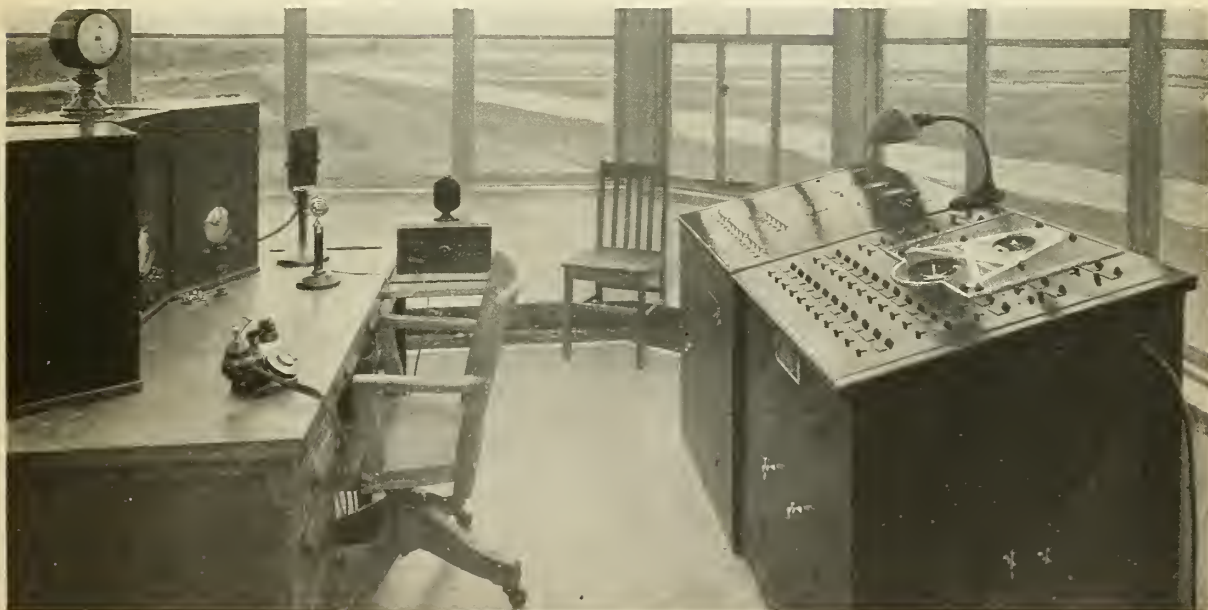
Lighting control desk (right) and radio equipment (left) in the control tower at Shushan Airport
